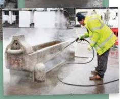
The trough was also cleaned using a fine jet of water at high pressure.
