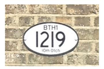
'BTH1' is the Engineer's Line Reference, which identifies the section of track, which is *South Bermondsey Junction to Sutton (East) Junction*, with the terminus being London Bridge station. The number 1219 identifies this bridge.
