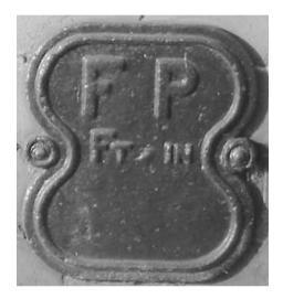
'F P' meant 'Fire Plug', an older name for a fire hydrant. The distance from the plaque to the hydrant is shown underneath in feet, and the size of the water pipe in inches.
