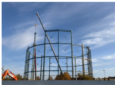
Demolition of the locally listed gasometer at Mitcham Gasworks – during a year when Merton Council unilaterally rewrote the site’s planning rules and there was minimal public engagement by tower blocks developer St William
