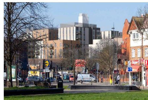
Proposed development for Mitcham Gasworks was universally condemned
